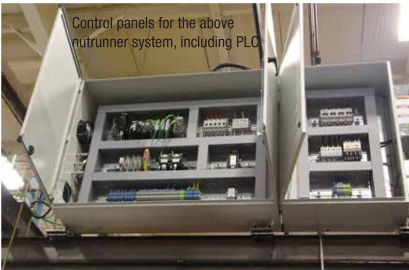
Control panels for the above nutrunner system, including PLC
